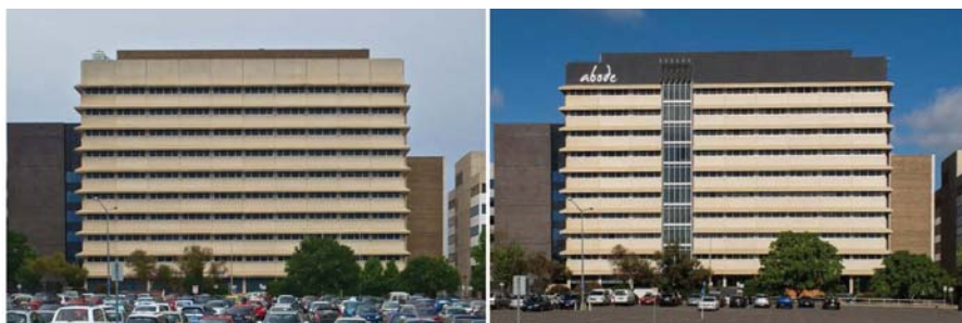
Abode the Apartment Hotel (Adaptive Reuse of Juliana House - before and after)
